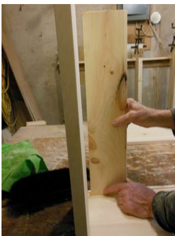
First board goes into dados on end and side
