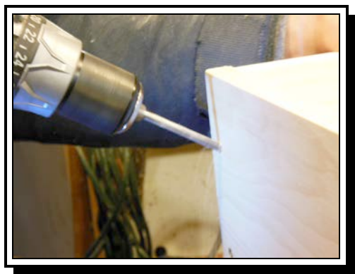
Drill new hole at 20° angle
