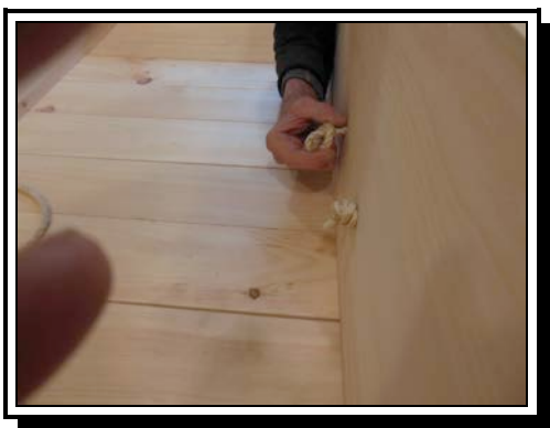
Thread rope from inside out then back in again. Tie knot #2
