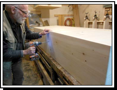
Drill hole part way through from outside
