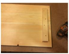
Line up the top boards (under side up), then screw the top cleats to the boards. The cleat is centered between the side edges and about 1 5/16" from the end of the boards. Screw the third cleat in the middle of the coffin top.
