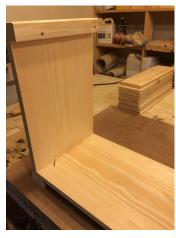
Stand end assembly upright with the wide side of corner board showing on the inside, set side boards on corner boards and screw into place with 1 1/4" screws.
