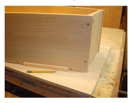
Set the assembled coffin on the top board. Using a one-half inch thick piece of wood, draw a line around the coffin. Saw along that line, then plane the edges smooth.
